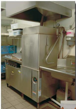
Vanguard's compact PowerMax 200™ Gas Booster Heaters (shown under dish table at left) consistently and reliably provide all the 125°F domestic hot water needs for the Marché Restaurant units as well as the 180°F sterilizing rinse water for the dishmachines. At that high temperature, dishware is sanitized without the need for harsh and costly chemicals, prolonging dishware life and producing a much cleaner outcome.
